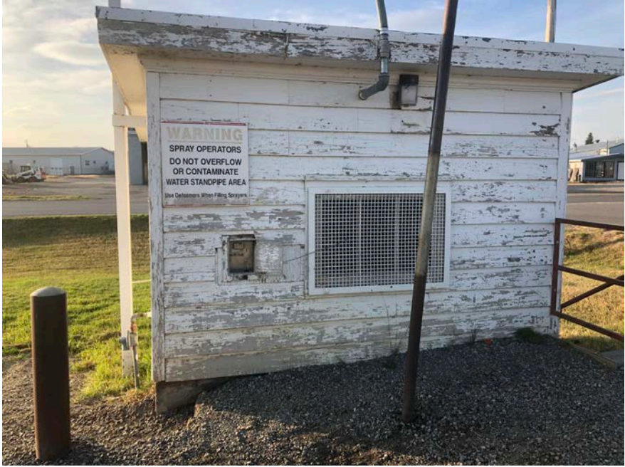
Site Photograph 2: Represents the Cowley standpipe.
